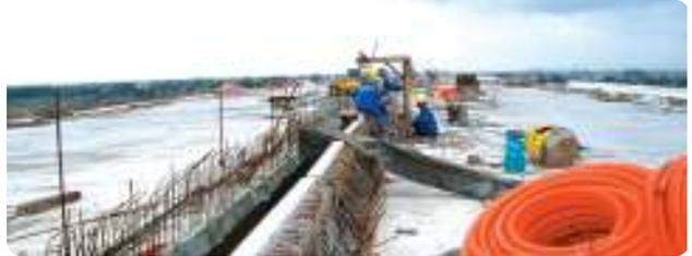
Cable installations on bridges or embedded in concrete with a space limited by its structure.
